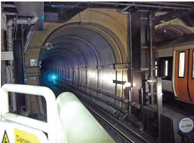
Southbound tunnel portal at Wapping
